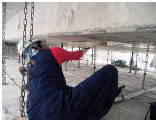
Applied on the floorboards.
