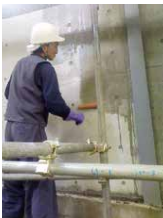
Applied with a roller
