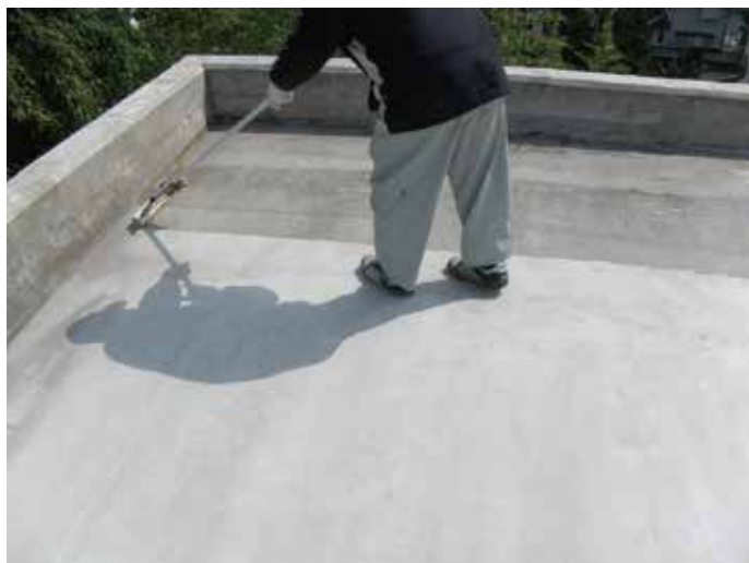
Repair cracks and joints before applying Ultratect WR. Use Ultratect CR for crack repairs.
