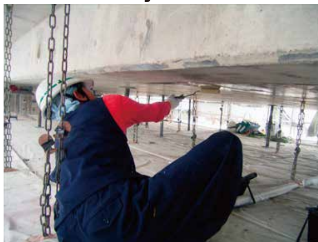
Applied to the underside of bridge slabs for waterproofing
