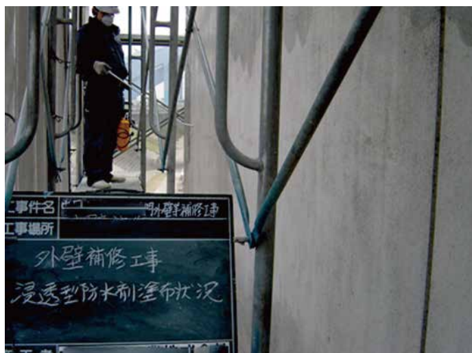
For waterproofing, anti-mold, and anti-fouling of concrete walls
